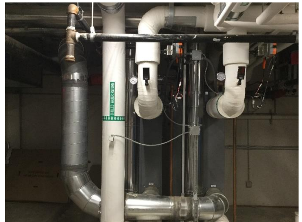
Building B Equipment Start-Up
