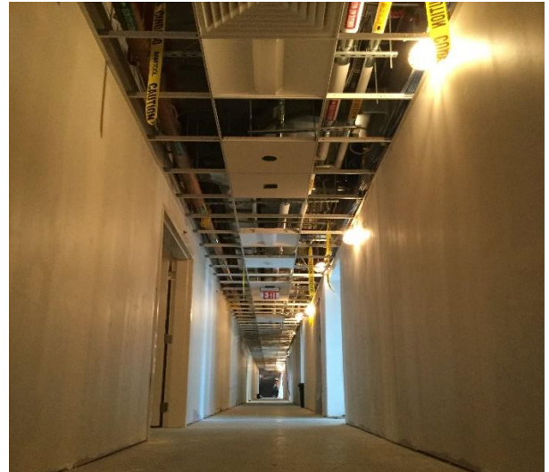
CL1 Corridor Overhead Rough-in
