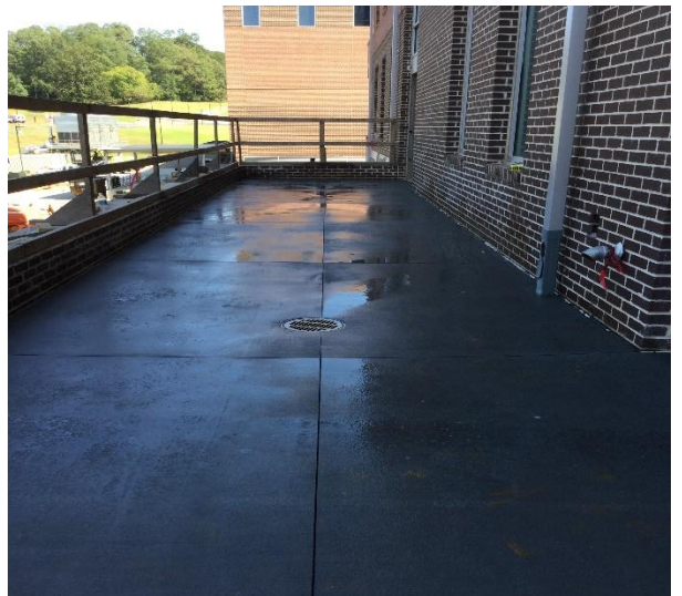
Building D Hardscape Placement
