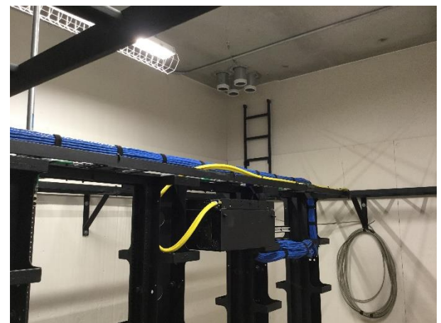
Building B Telecom Room Buildout
