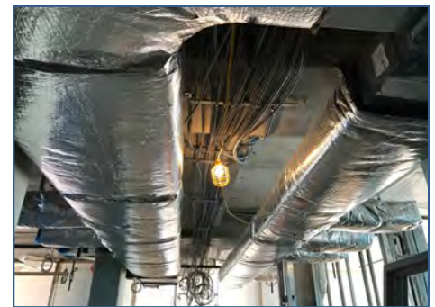
Building B Duct Insulation
