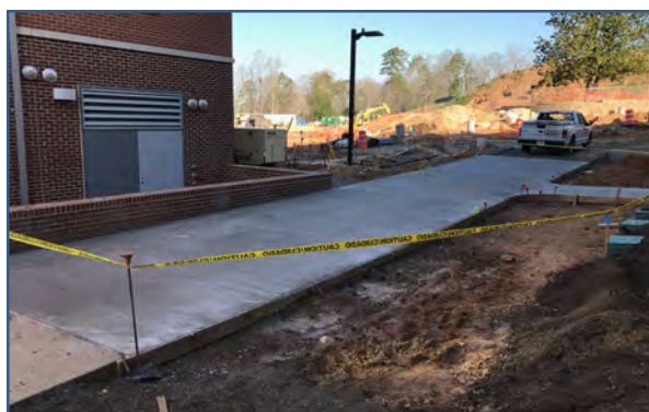
Fire Lane Between Bldgs. E & F
