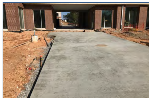
Fire Lane & Building E Breezeway
