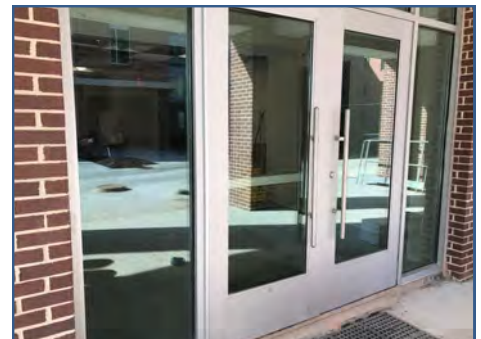
Building F Exterior Door Hardware Installed
