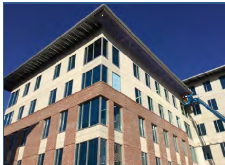
Bldg. B DEFS Board
