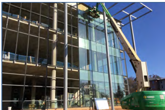
HUB Curtain Wall
