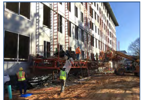
Bldg. C Brick Masonry
