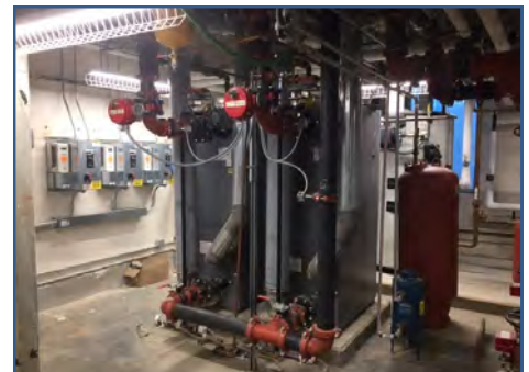
Bldg. G Mech. Room
