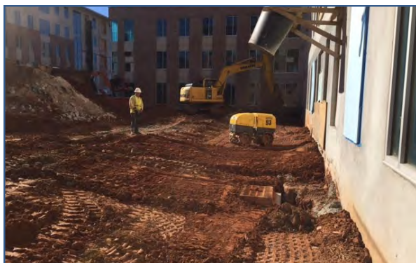
Storm Drains @ Bldg. B
