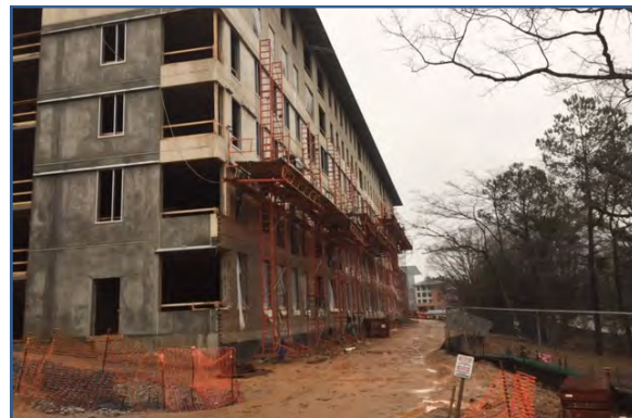
Bldg. C Brick @ South Side
