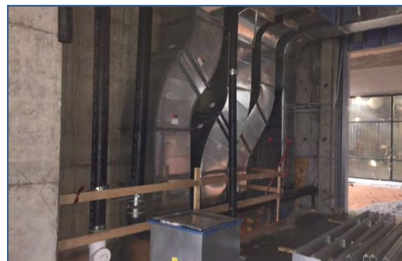
Duct Shaft Rough-in @ HUB
