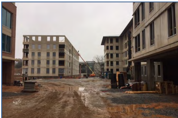
Precast Complete/Crane Gone
