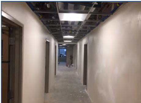
Finishing Corridors @ Bldg. E
