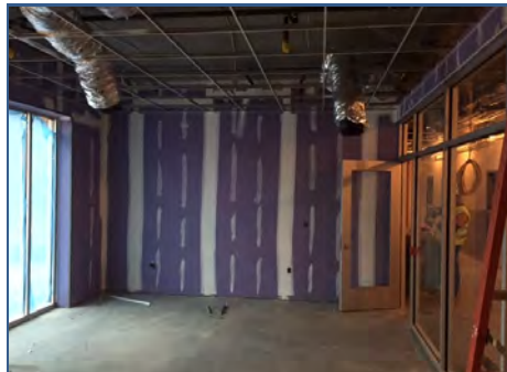
Bedding & Taping @ Bldg. E
