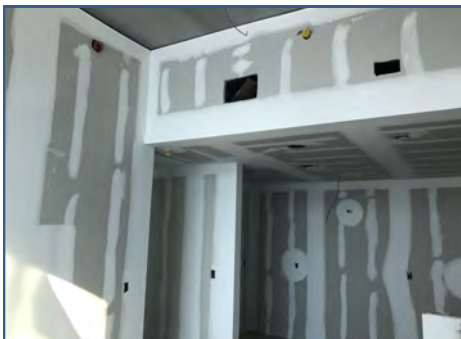
Bedding & Taping @ Bldg. A
