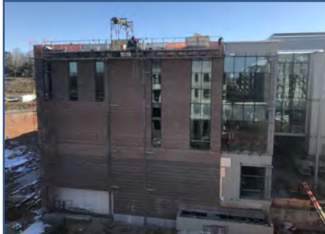
HUB Masonry - West Elevation
