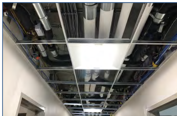
Corridor Lights @ Building G
