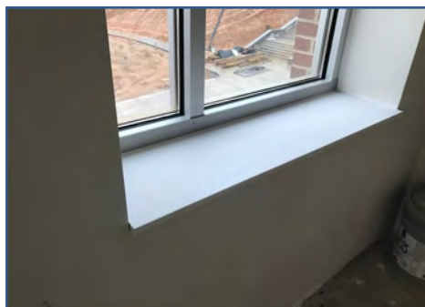
Bldg. G Window Sill
