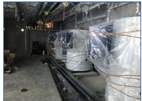
Building B - Mechanical Room
