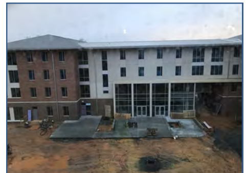
Bldg. E Terrace
