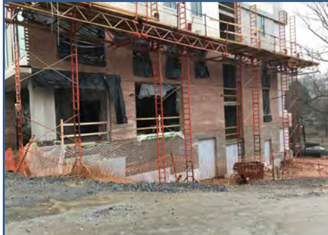
Building C Masonry- West Elevation
