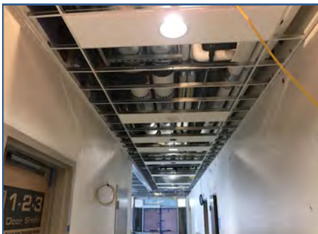
Building G 1st Floor Corridor Lights
