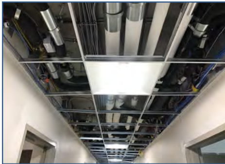
Bldg. G Light Fixtures and Ceiling Grid
