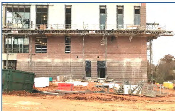
HUB Brick – East Wall
