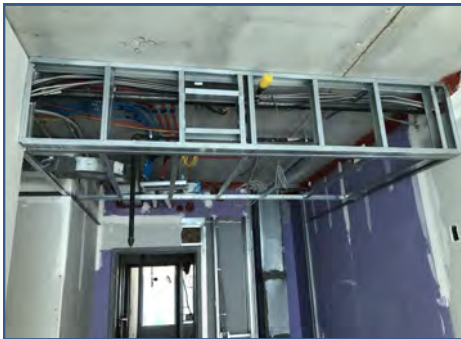
Bldg. A Interior Soffit Framing
