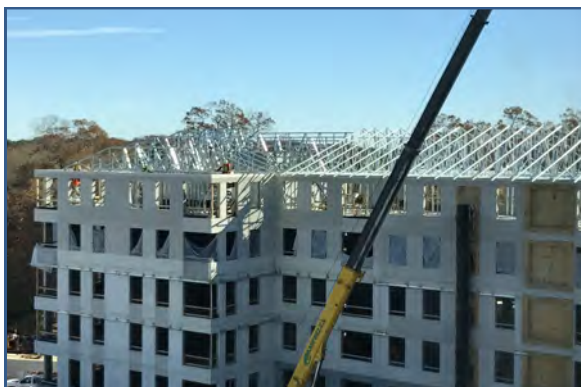
Bldg. C Roof Trusses
