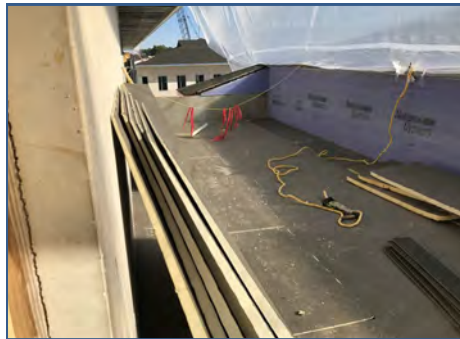
Bldg. B Flat Roof
