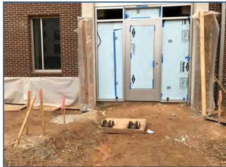
Bldg. F Storefront Doors
