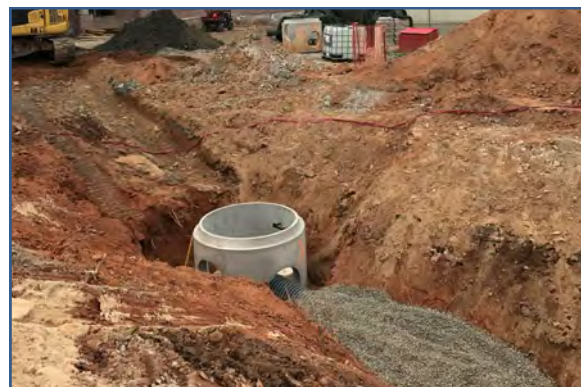
Storm Line - West Of Building B
