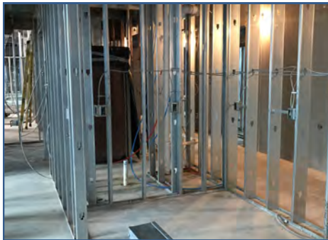
Bldg. B Interior Framing
