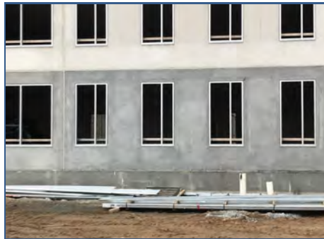
Bldg. C Window Frames
