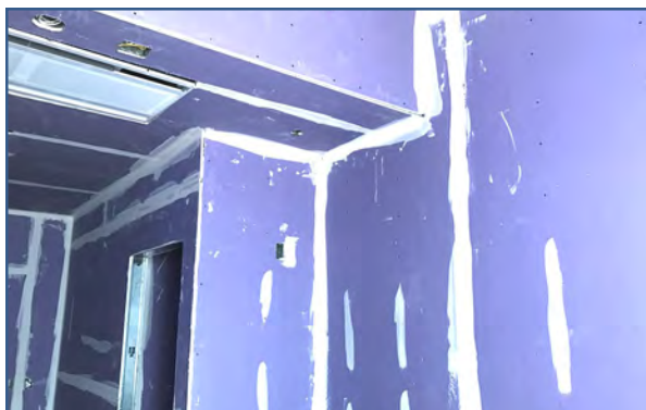
Building E Finishing
