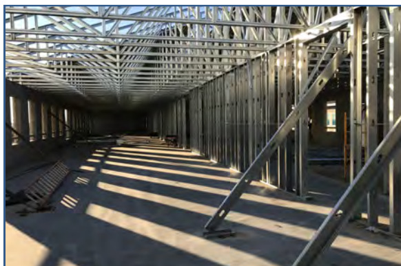
Bldg. C Roof Trusses & Load Bearing Walls
