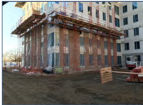
Bldg. B West Wing Brick
