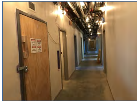
Bldg. F 1st Floor Painting
