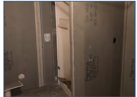
Bldg. E Showers
