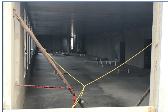
Building D SOG
