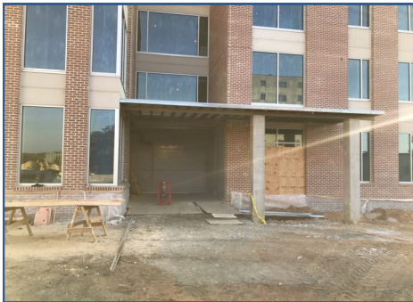
Bldg. A Flat Roof
