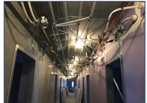
Bldg. E 3rd Floor Rough-In
