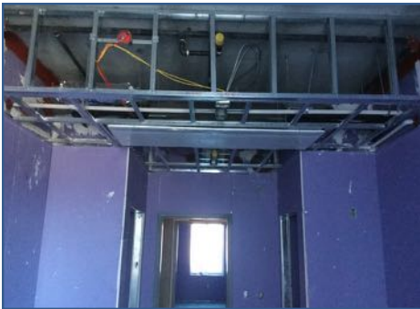
Bldg. E Interior Soffit Framing
