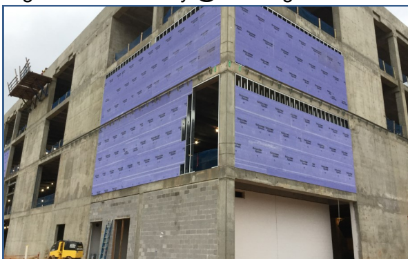
HUB Exterior Wall Framing
