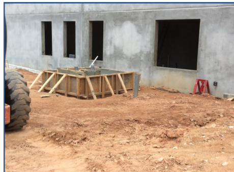
Bldg. B Transformer Pad
