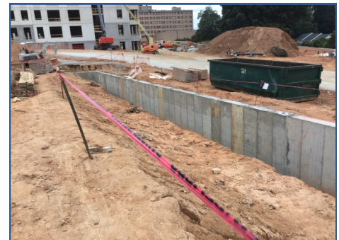
Bldg. D CIP Walls
