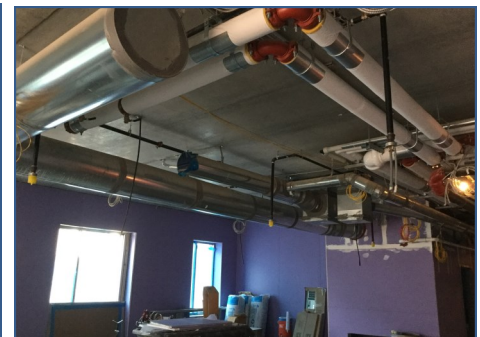
Bldg. F Overhead Rough-In
