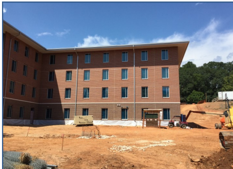
Bldg. G Downspouts
