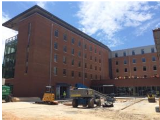
North East - Bldg. A
