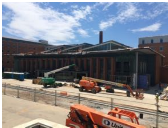
East - Bldg. B
