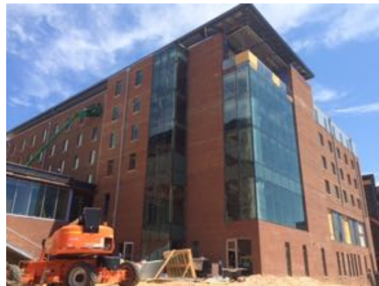
North West - Bldg. C
