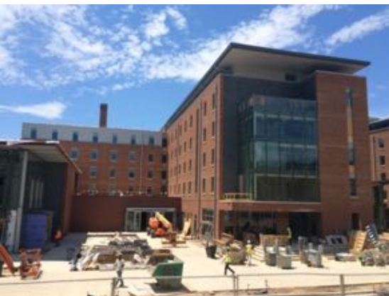
South East - Bldg. C
