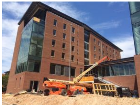
South West - Bldg. D
