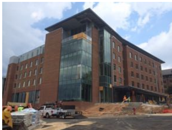
South West - Bldg. A
