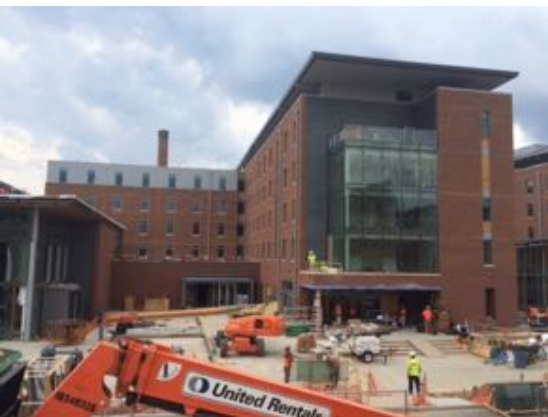
South East - Bldg. C
