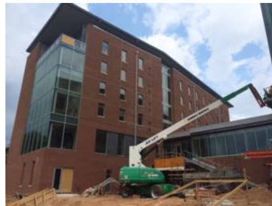
South West - Bldg. D
