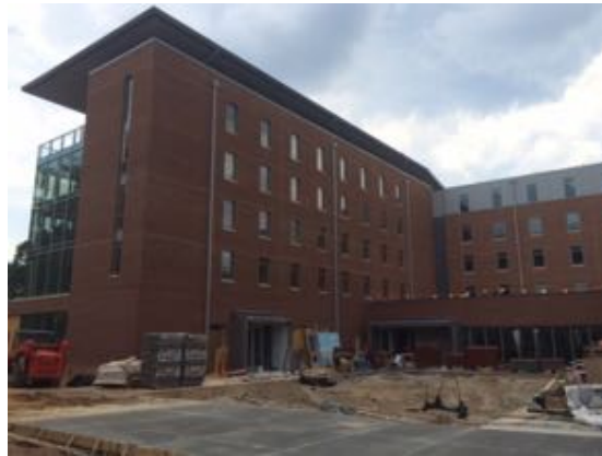
North East - Bldg. A
