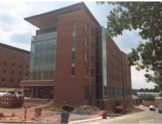
North East - Bldg. D
