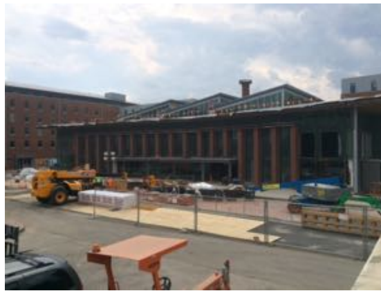
East - Bldg. B
