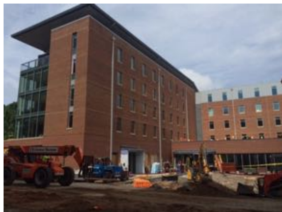
North East - Bldg. A
