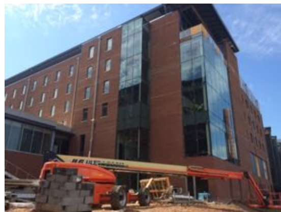
North West - Bldg. C
