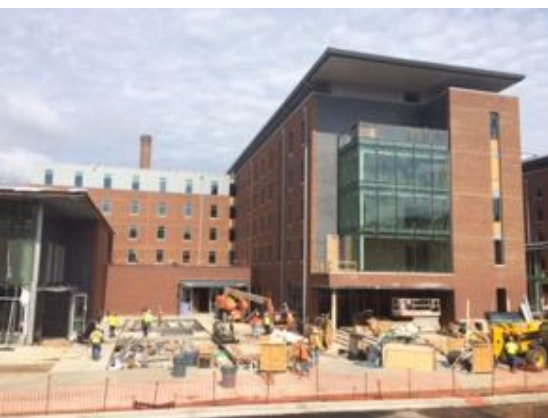
South East - Bldg. C
