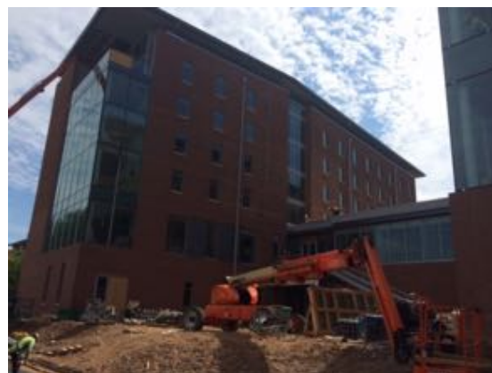
South West - Bldg. D
