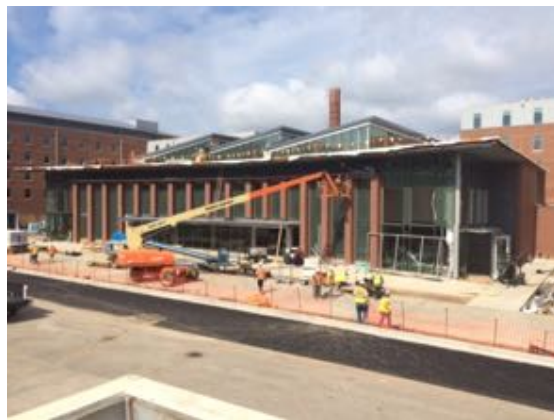
East - Bldg. B
