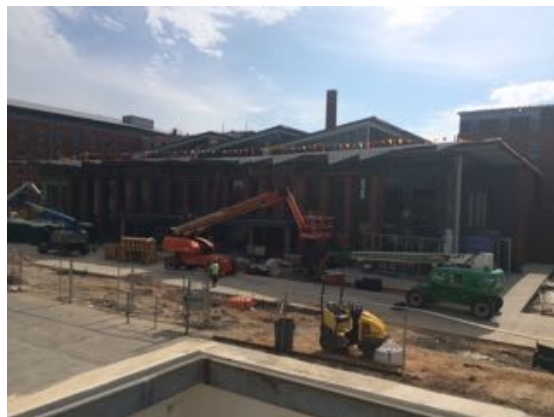
East - Bldg. B
