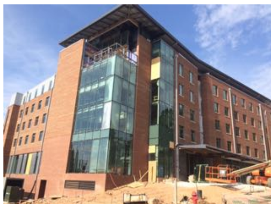
South West - Bldg. A
