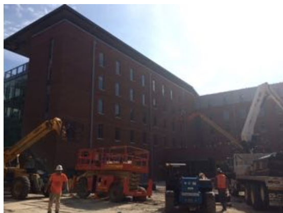
North East - Bldg. A
