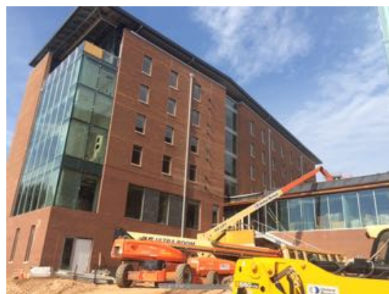
South West - Bldg. D
