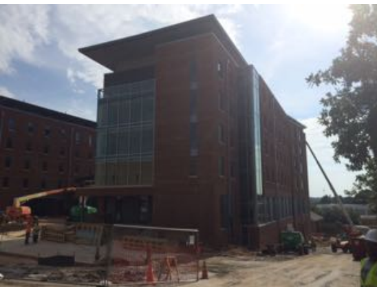
North East - Bldg. D
