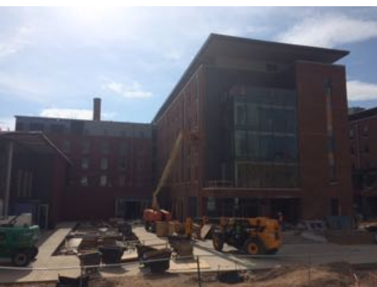
South East - Bldg. C
