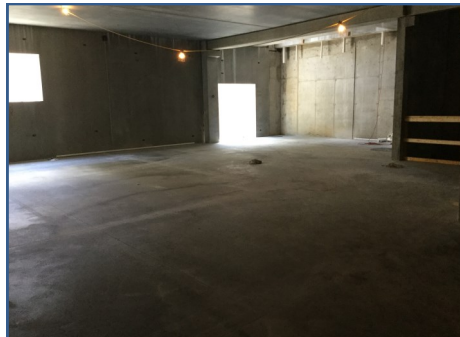
Bldg. E Basement SOG
