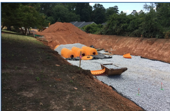
Chambers at Underground Detention
