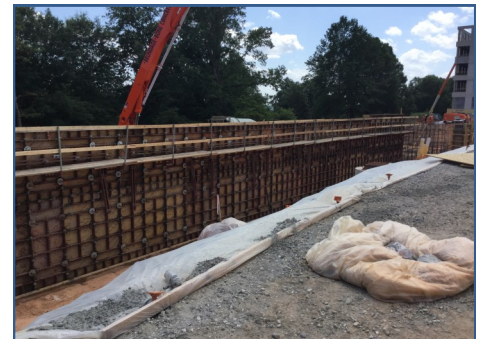
Bldg. C CIP Walls
