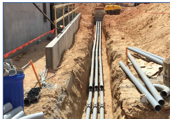
Building B Ductbank to Transformer
