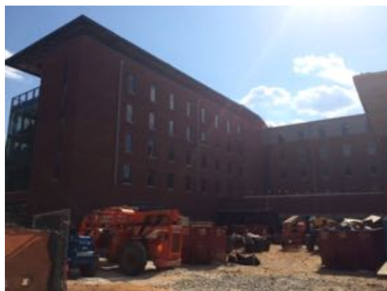
North East - Bldg. A
