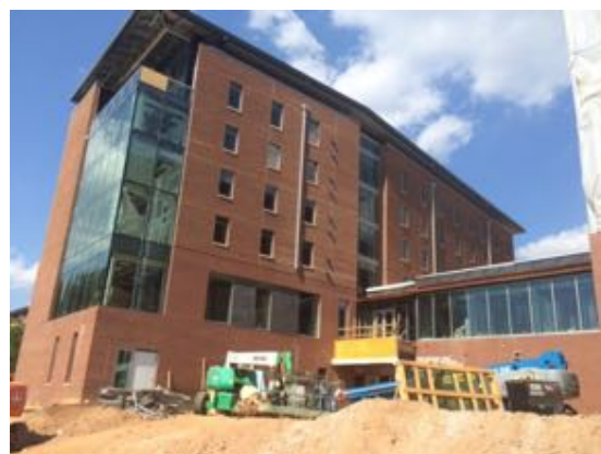
South West - Bldg. D
