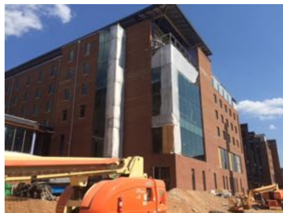
North West - Bldg. C
