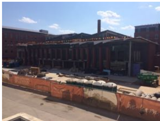
East - Bldg. B
