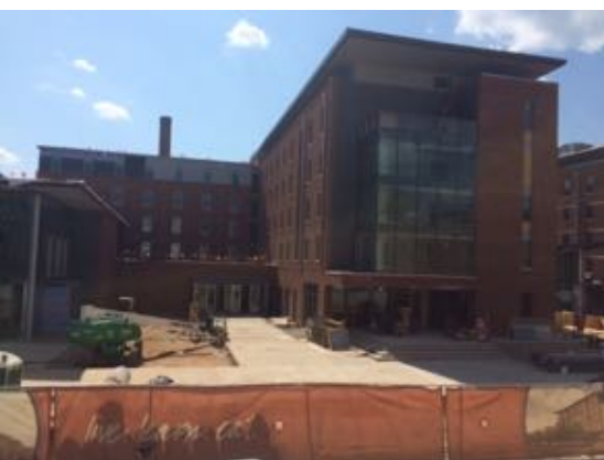
South East - Bldg. C
