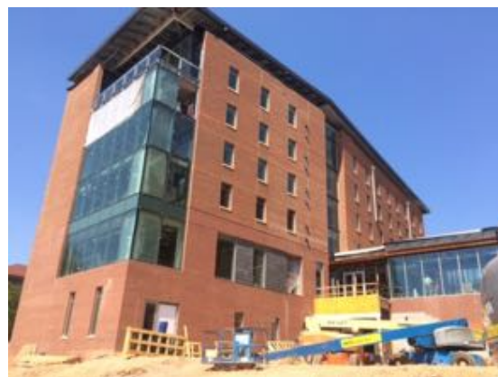
South West - Bldg. D
