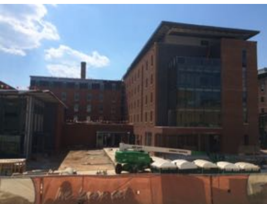
South East - Bldg. C
