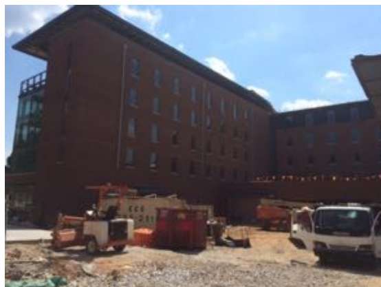
North East - Bldg. A
