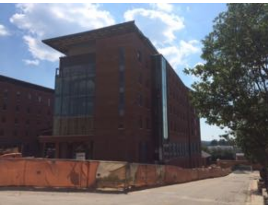
North East - Bldg. D
