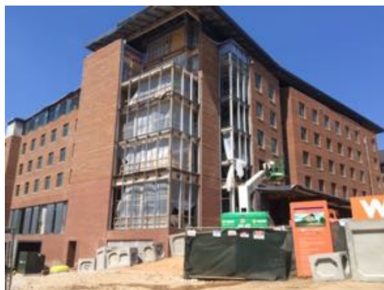
South West - Bldg. A
