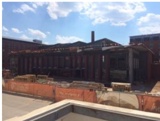
East - Bldg. B
