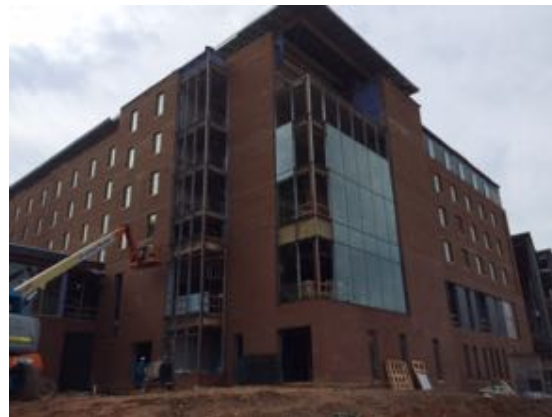
North West - Bldg. C
