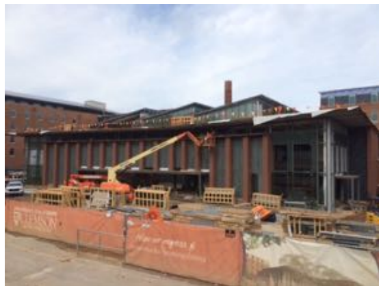
East - Bldg. B
