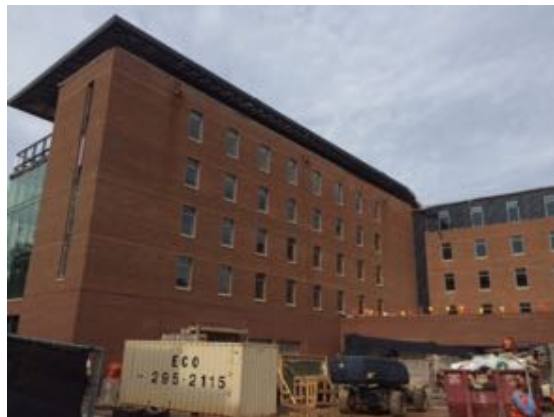
North East - Bldg. A
