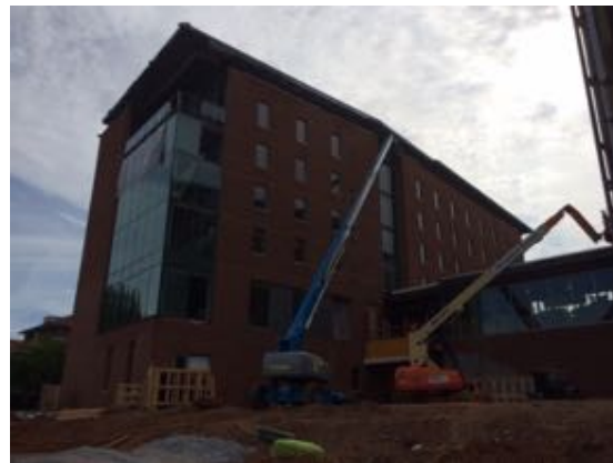
South West - Bldg. D
