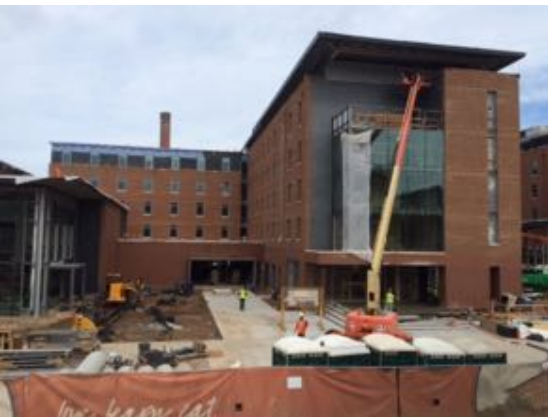
South East - Bldg. C
