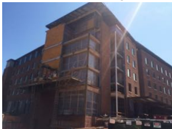
South West - Bldg. A
