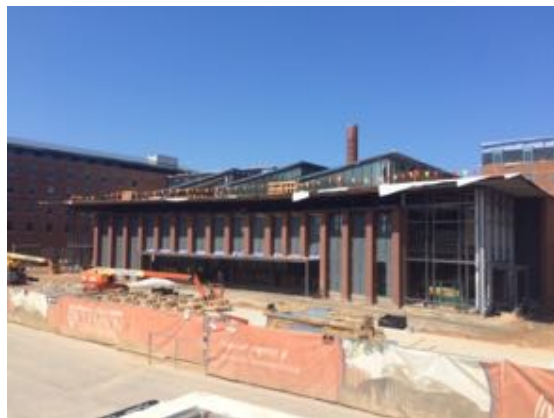
East - Bldg. B
