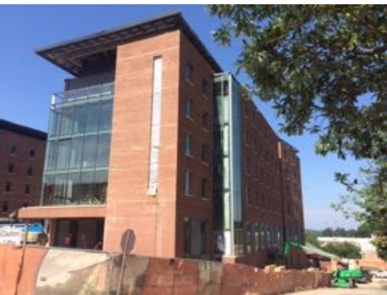
North East - Bldg. D
