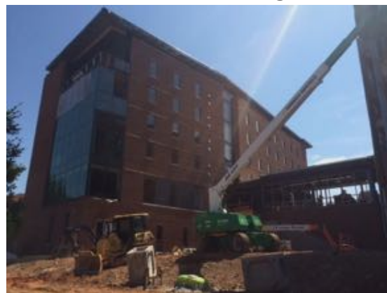
South West - Bldg. D
