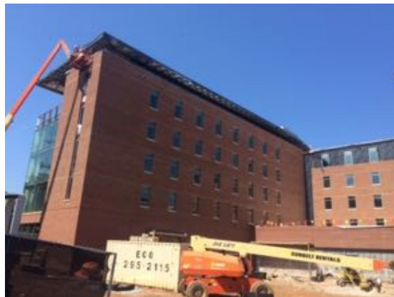
North East - Bldg. A
