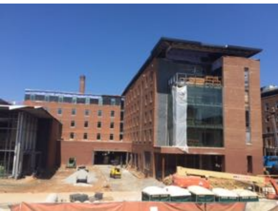
South East - Bldg. C
