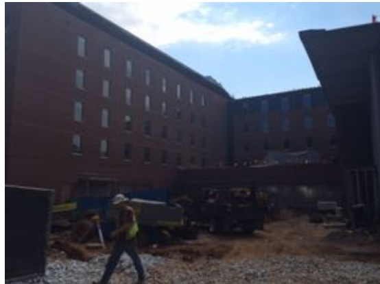
North East - Bldg. A
