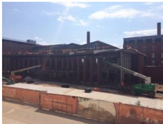
East - Bldg. B
