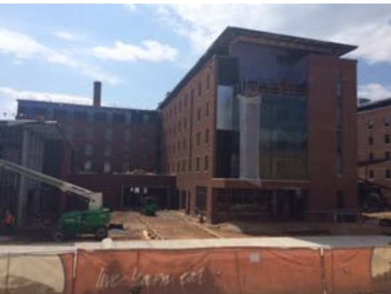
South East - Bldg. C
