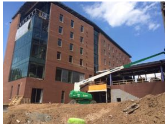
South West - Bldg. D
