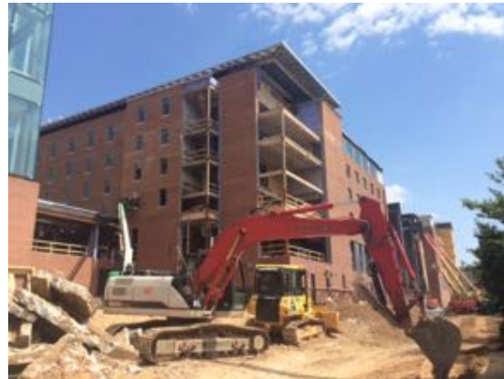
North West - Bldg. C
