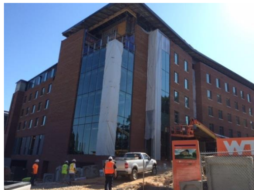
South West - Bldg. A
