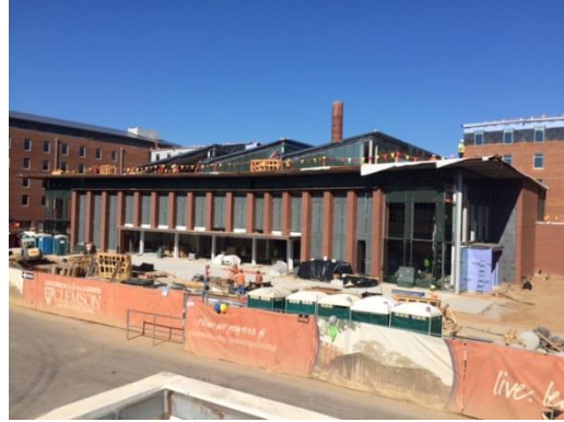
East - Bldg. B
