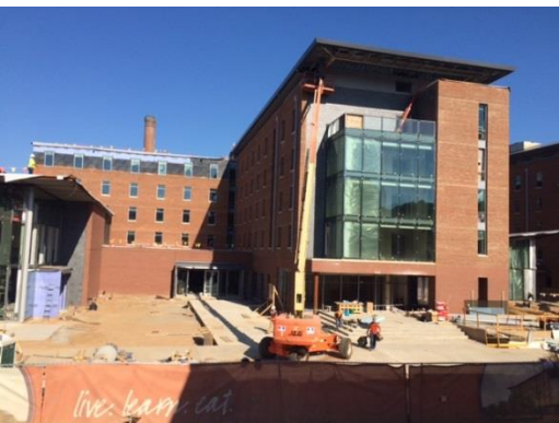
South East - Bldg. C
