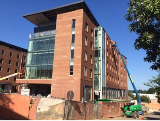
North East - Bldg. D
