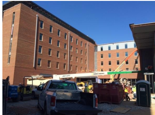
North East - Bldg. A
