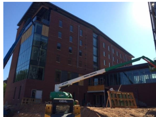
South West - Bldg. D
