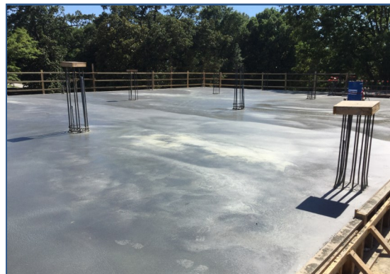
HUB Elevated Slab 2C
