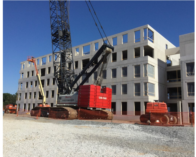
Building A Precast
