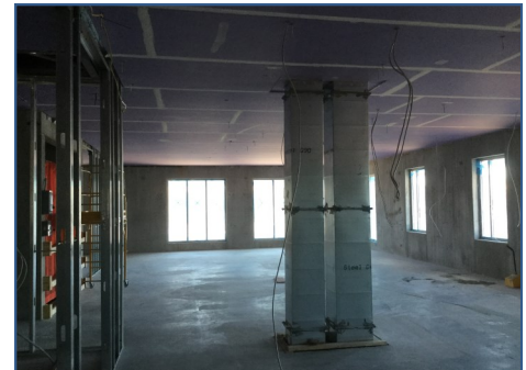
Bldg. F Ceiling Install & Overhead Rough-In.
