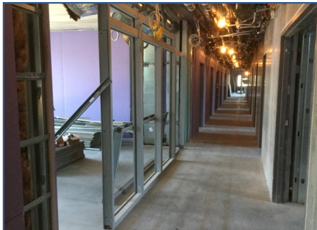
Bldg. G Fire Rated Storefront Assembly
