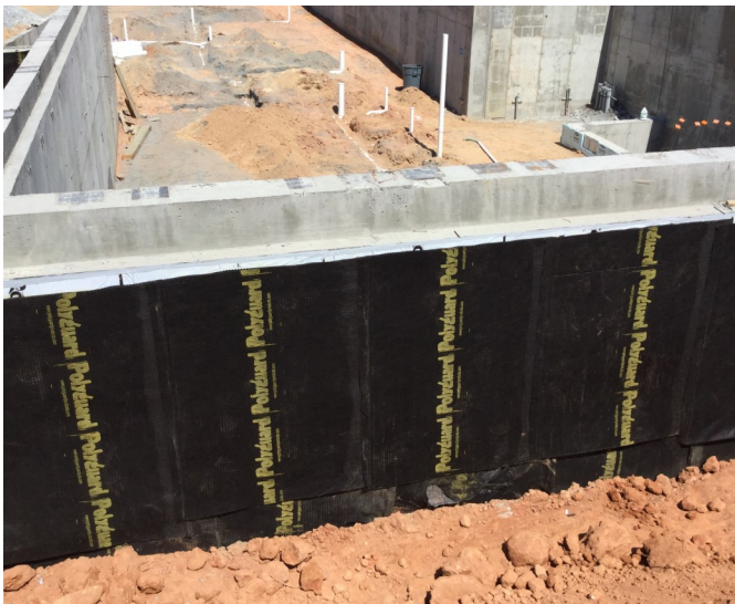
Building B Waterproofing
