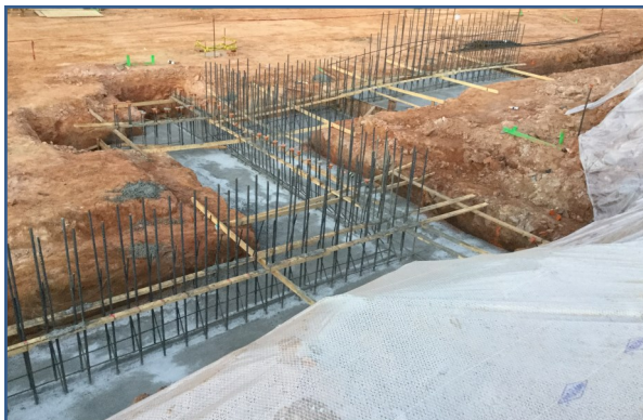
Building C Footings
