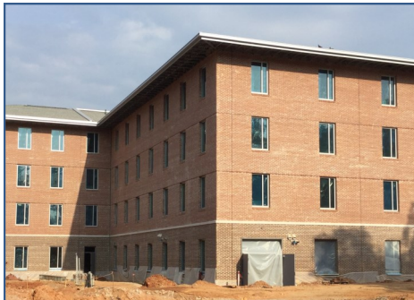
Bldg. G Brick
