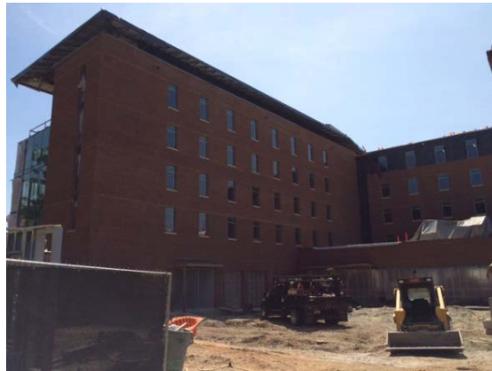
North East - Bldg. A
