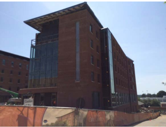
North East - Bldg. D
