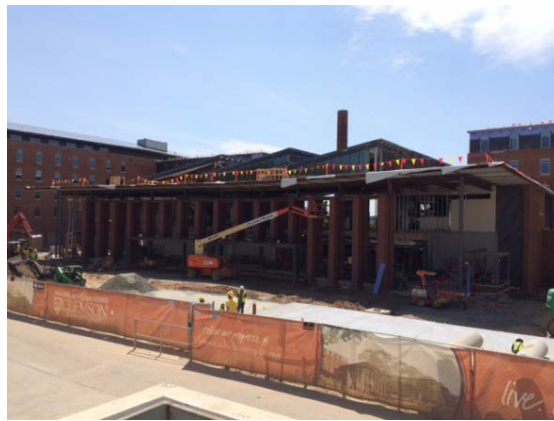
East - Bldg. B
