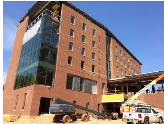
South West - Bldg. D
