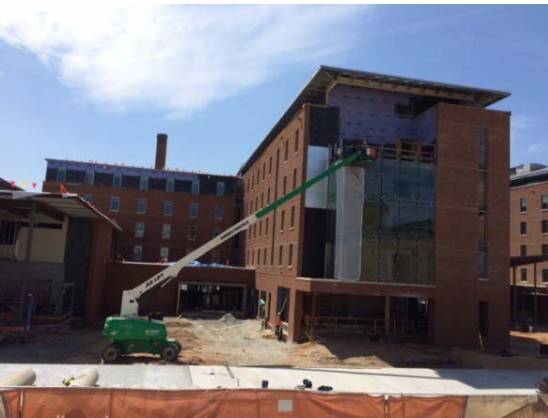
South East - Bldg. C
