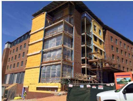
South West - Bldg. A
