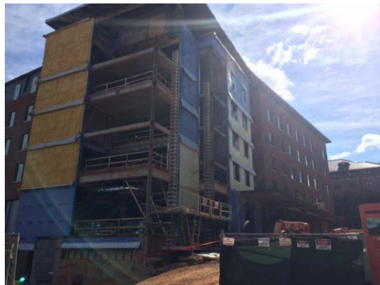
South West - Bldg. A
