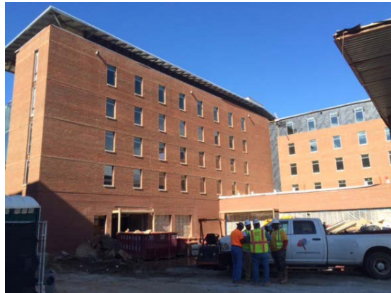
North East - Bldg. A
