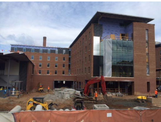
South East - Bldg. C
