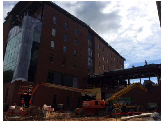
South West - Bldg. D
