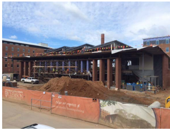
East - Bldg. B
