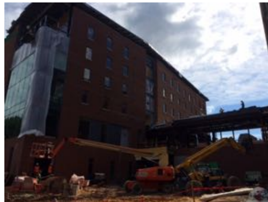
South West - Bldg. D
