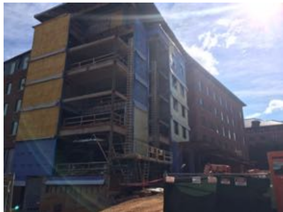
South West - Bldg. A
