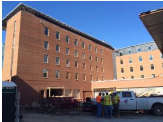
North East - Bldg. A
