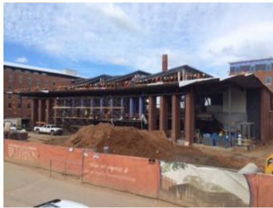
East - Bldg. B
