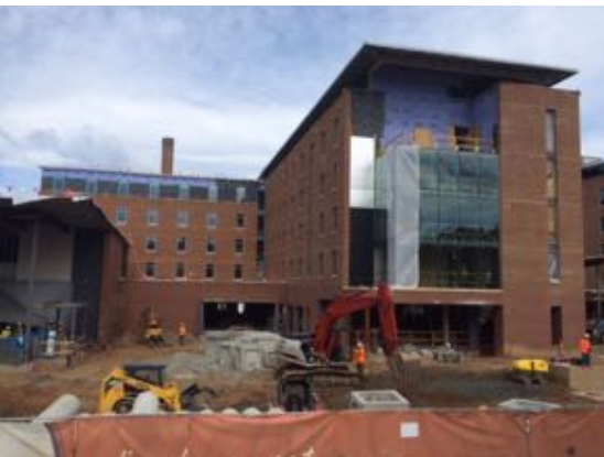
South East - Bldg. C
