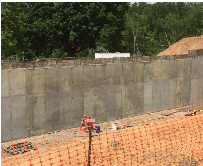
Building B CIP Walls
