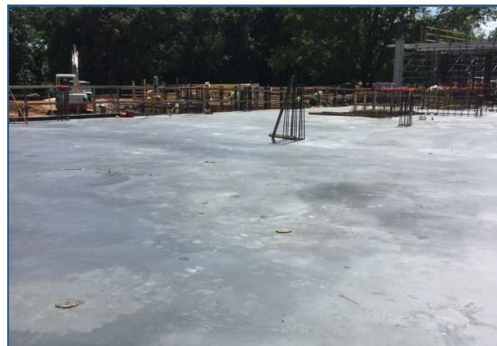
Elevated Slab 1B @ HUB
