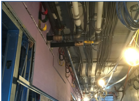
Bldg. G Chilled Water
