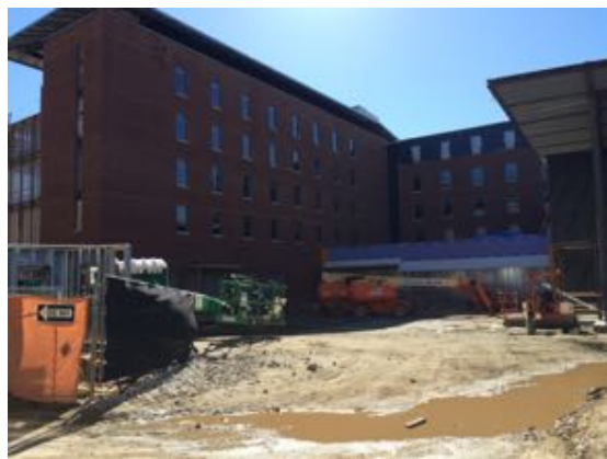
North East - Bldg. A
