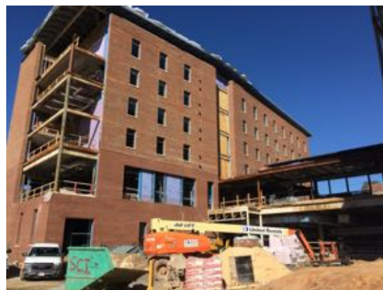
South West - Bldg. D
