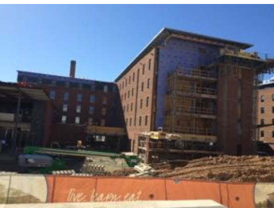
South East - Bldg. C
