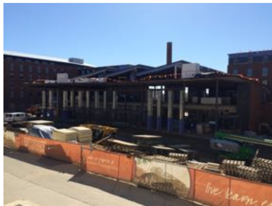
East - Bldg. B
