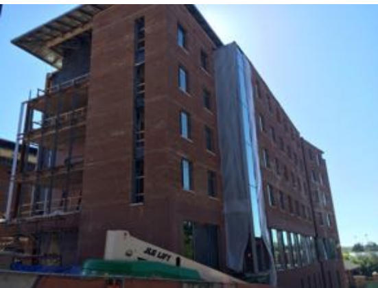
North East - Bldg. D
