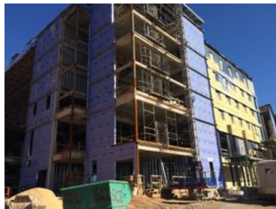
West - Bldg. C
