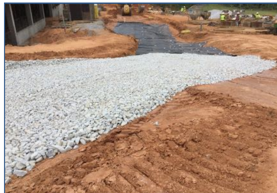
Access Road @ HUB
