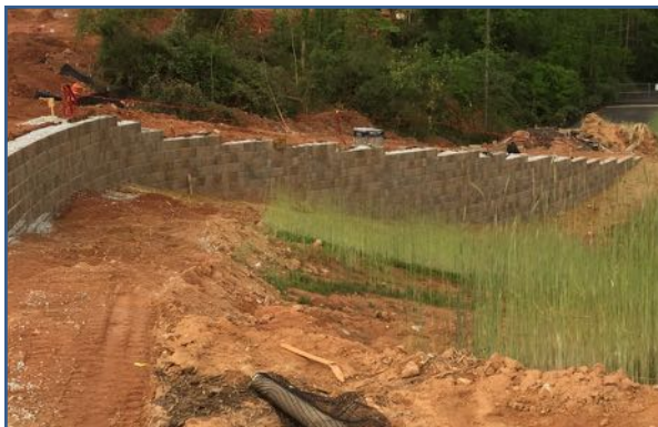
Retaining Wall @ HUB
