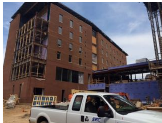
South West - Bldg. D
