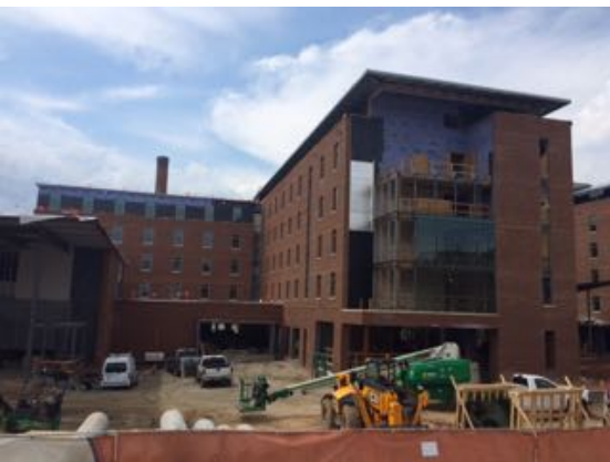
South East - Bldg. C
