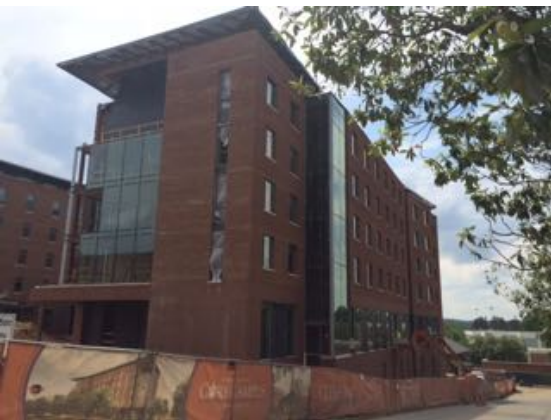
North East - Bldg. D
