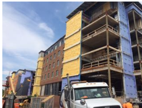
West - Bldg. A & B
