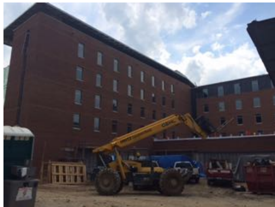
North East - Bldg. A
