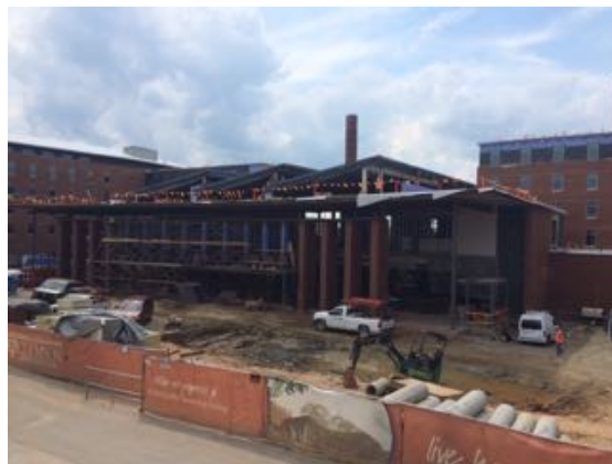
East - Bldg. B
