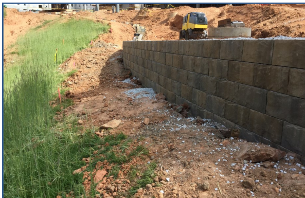
Retaining Wall @ HUB
