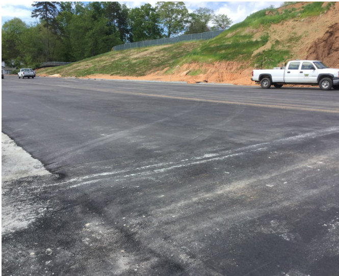
Paving @ NW Parking Lot
