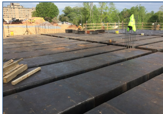
Elevated Deck @ HUB
