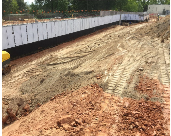
Building A Backfill
