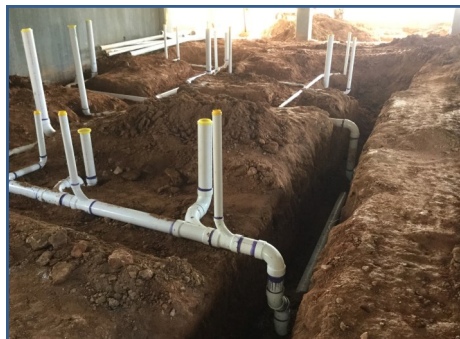
Bldg. E Plumbing
