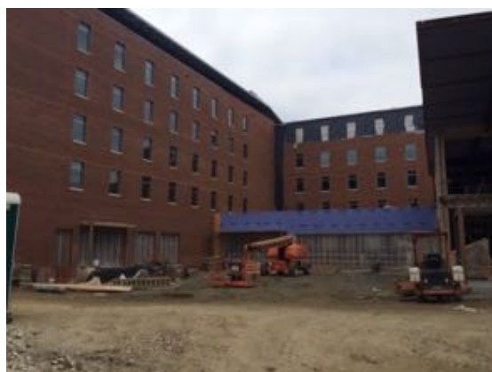
North East - Bldg. A
