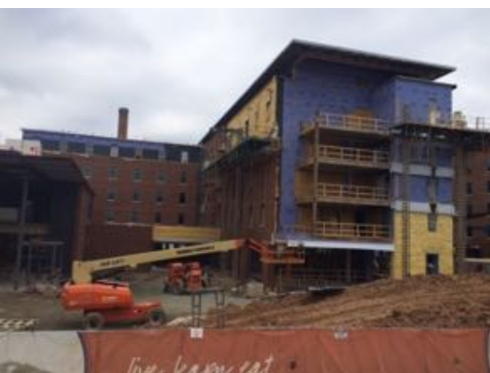
South East - Bldg. C
