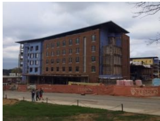
South East - Bldg. A
