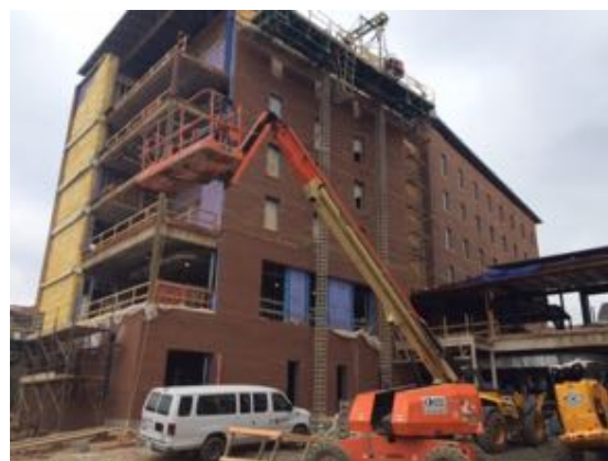
South West - Bldg. D
