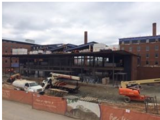
East - Bldg. B
