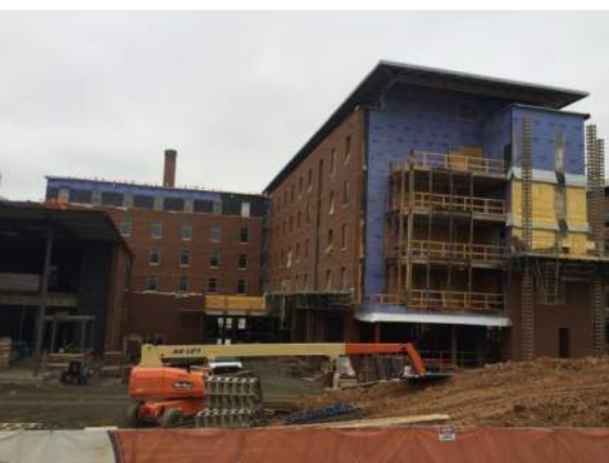
South East - Bldg. C
