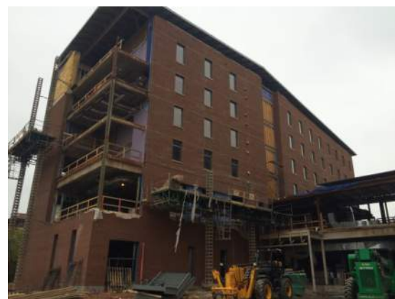
South West - Bldg. D
