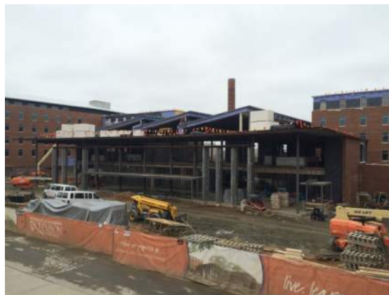
East - Bldg. B
