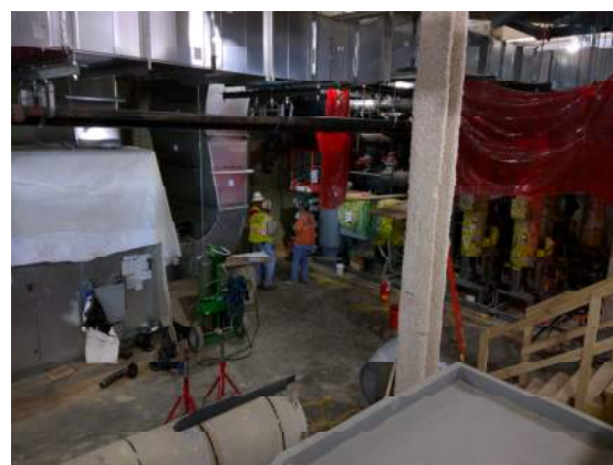
Bldg. D/C Mechanical Room
