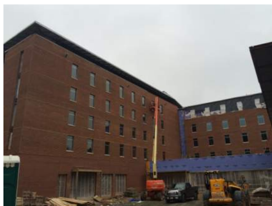
North East - Bldg. A
