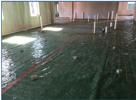
Bldg. G Slab on Grade Prep
