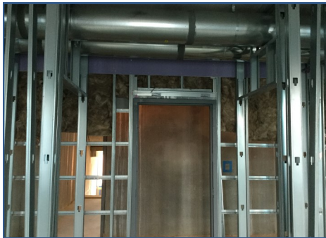
Bldg. G Hanger Duct
