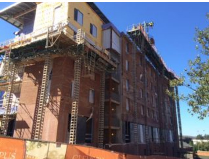
North East - Bldg. D
