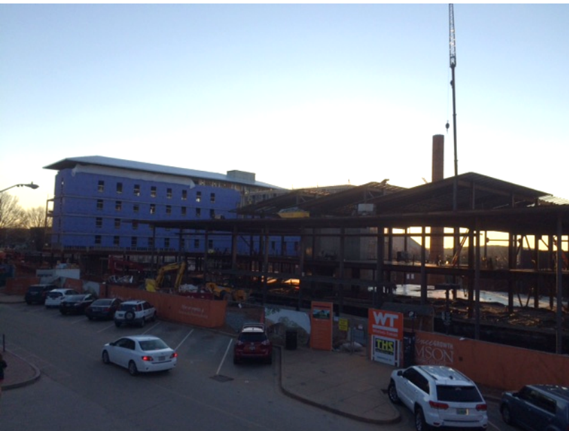
View of Building A & B
