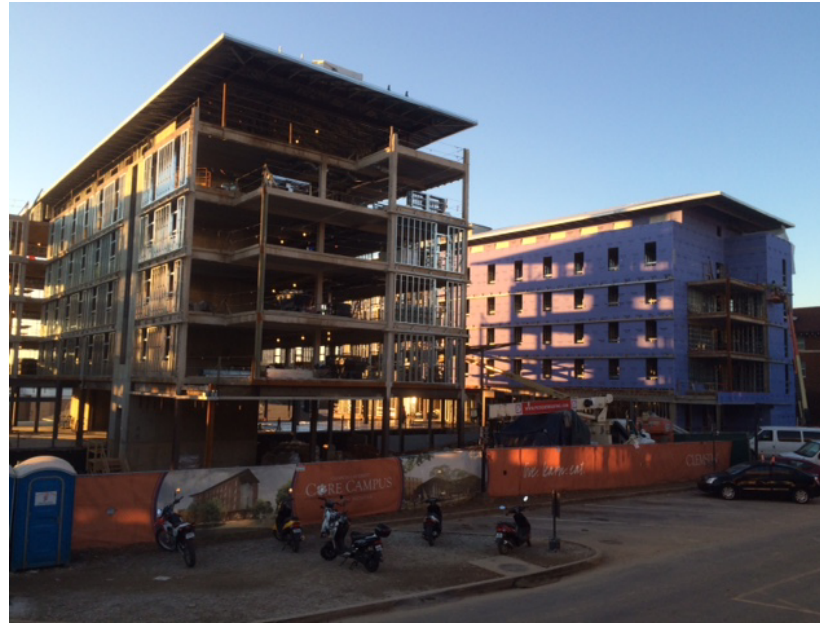
View of Building C & D
