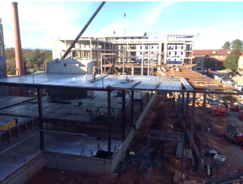
View of Building B & C
