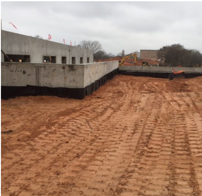
Building F Waterproofing & Backfill
