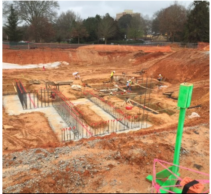
Foundations @ Building E
