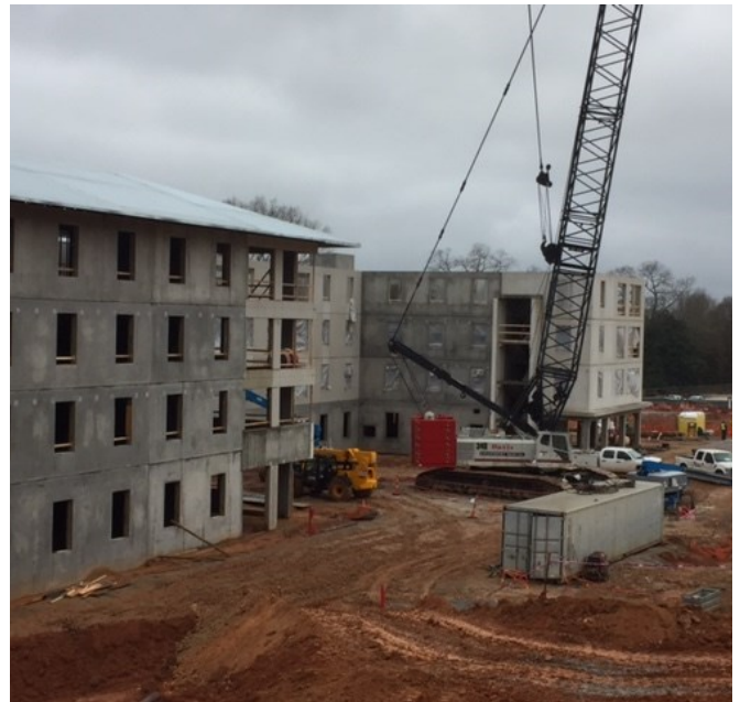
Roof Trusses/Decking at Building G
