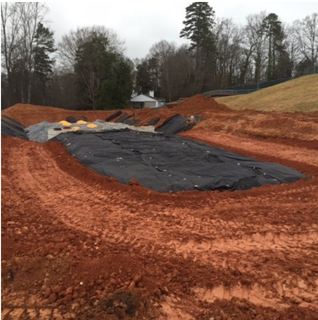
Underground Detention Tank
