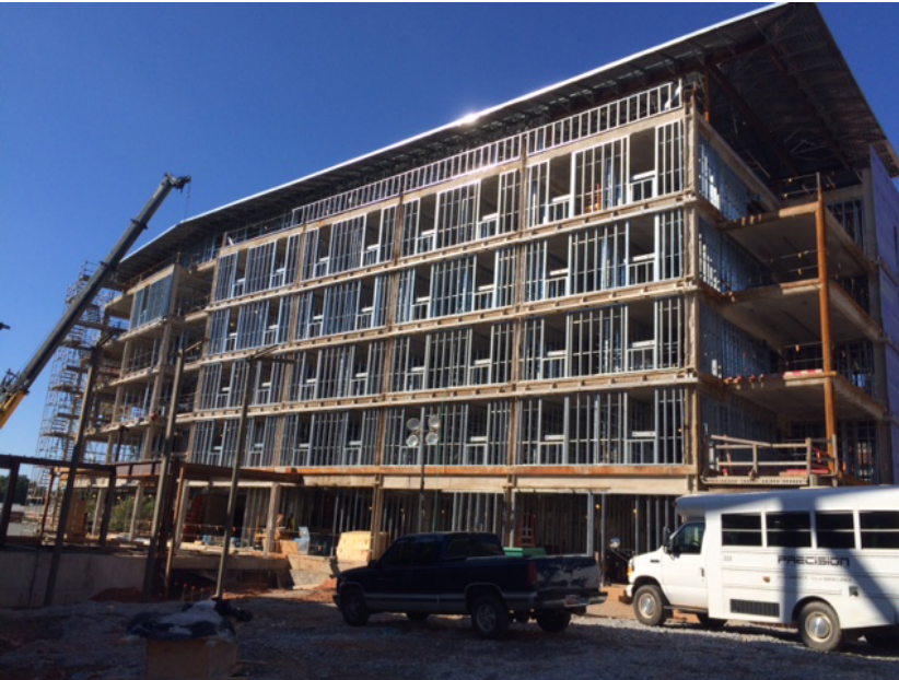
View of Building D
