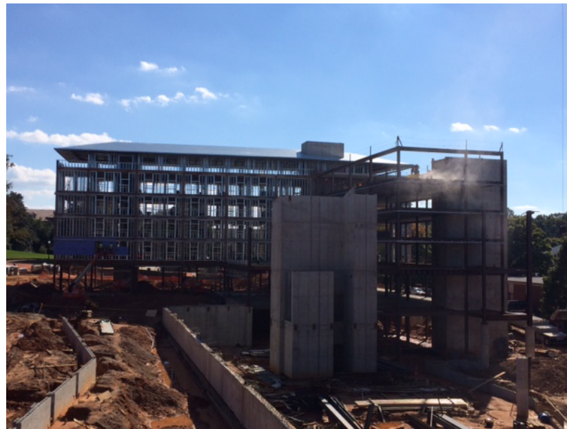
View of Building A & B
