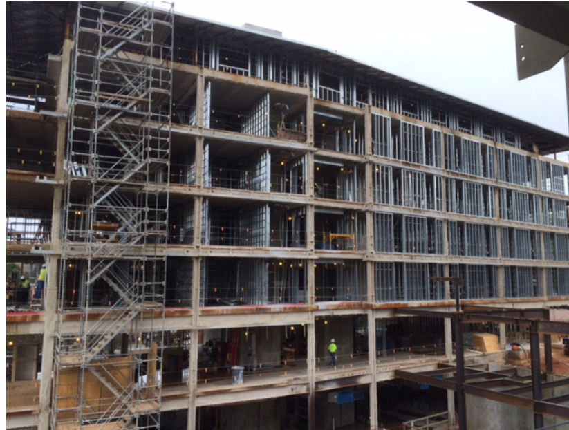
Building C View of Building D
