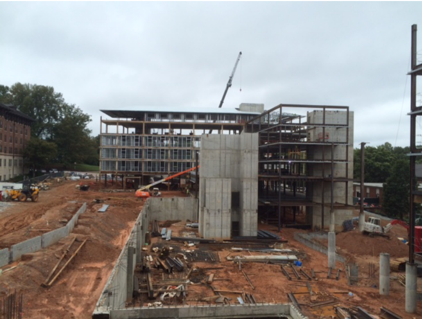
Building C View of Building A
