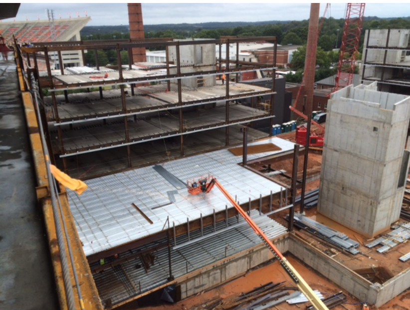
View of Building A and B
