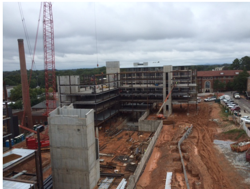
Building A View of Building C
