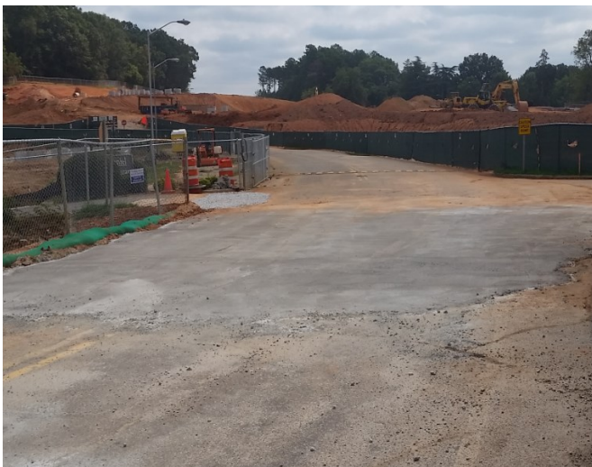
Concrete patching on Daniel Dr.
