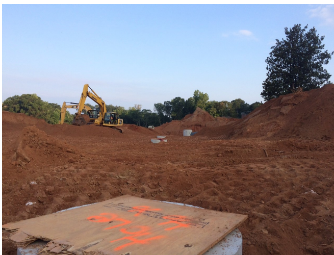
Storm Line #4A install
