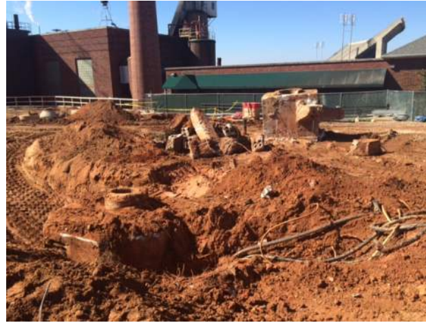
Duct Bank Demo
