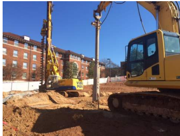
Aggregate Pier Install
