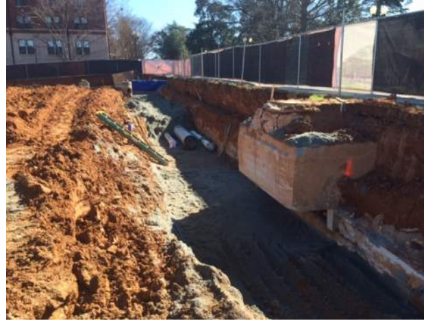
Steam Pipe Install
