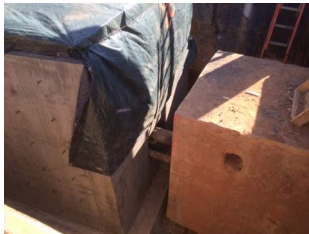
Concrete Steam Vault
