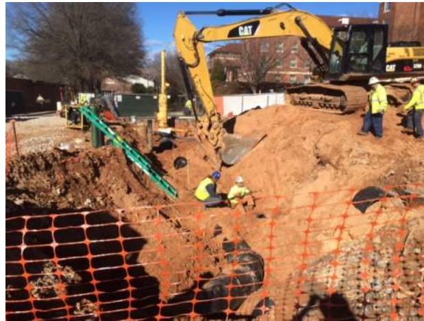
Chilled Water Tie-in
