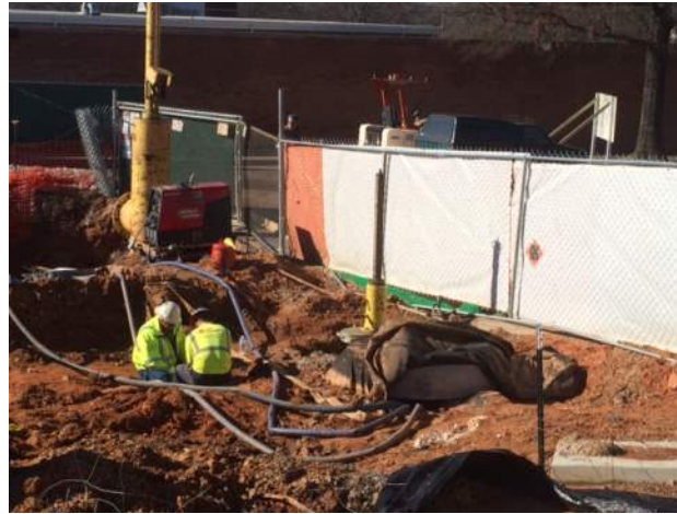
Water Line Stop
